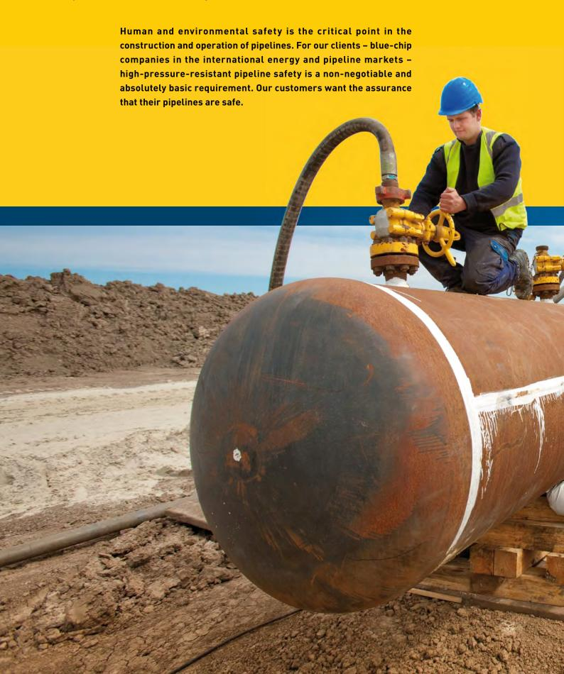
Non-destructive testing and reliable determination of guaranteed pressure resistance is the safety "passport" for pipeline construction. The tests of imperviousness and strength conducted by RAS using air, gas and water are our most important tasks in the pre-commissioning of pipelines.
